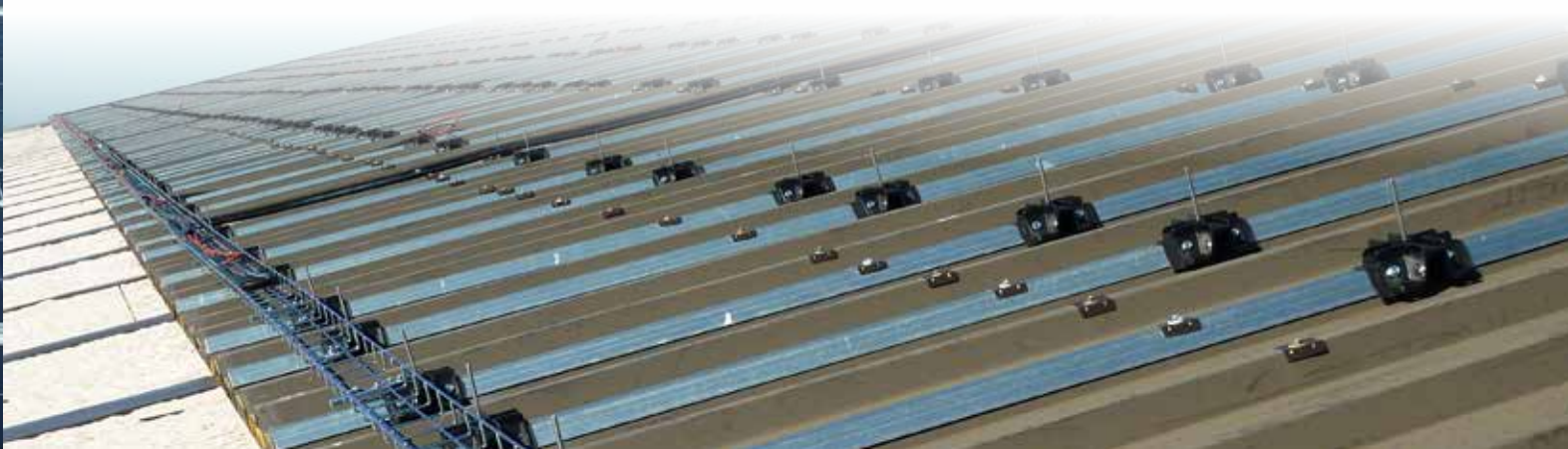
Fig. C - fixing with terminal plate To be used at beginning-end of the photovoltaic module row
